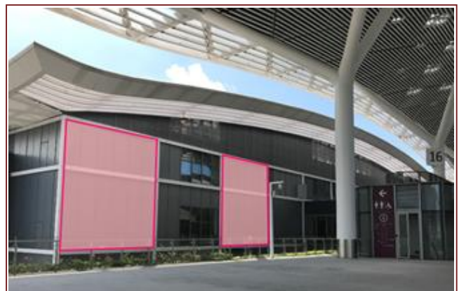
B03(b) Banner – Hall entrance (external): Central corridor (upper)
